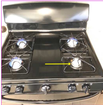
One or more rangetop burner igniters failed to ignite a gas burner.
